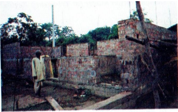
Ram Tilak and his house during construction
